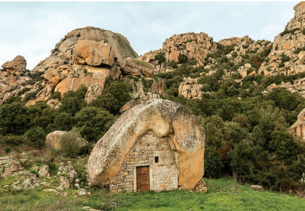
This rock hollowed out by erosion and walled up with stones was likely used by shepherds as a shelter near the historic Sardinian village of Tempio Pausania.
